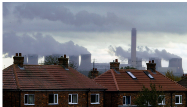
Figure 3 – Drax power station, the UK's largest coal-burning power station, has so far been the UK's largest burner of biomass. Both biomass and coal are heavy pollutants - yet air quality impacts of biomass are not addressed by any sustainability standards in the UK. IStock Photos
